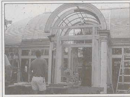
TIM REYNOLDS SURVEYS THE RECONSTRUCTION OF CONSERVATORY ENTRANCE, JULY 1995.
