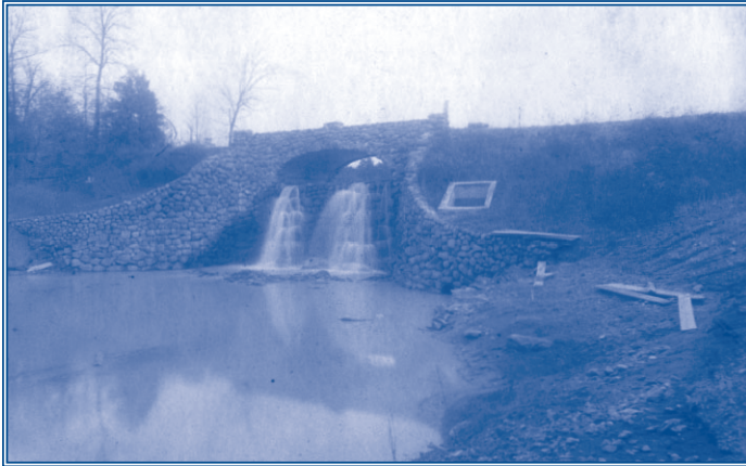
LANDSCAPE AROUND THE DAM UNDER CONSTRUCTION.
