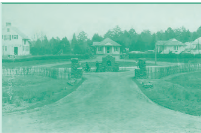
WALLS AND FOUNTAINS ARE ALMOST IDENTICAL TO FEATURES AT DUKE FARMS.
